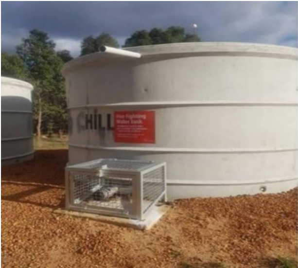
Strategic 47,000 Litre Concrete Tank & Protected Fittings
