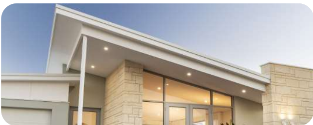
Plate 24 Image: Example of skillion roof at max height, with remaining built form heights lower (from colorbond)
