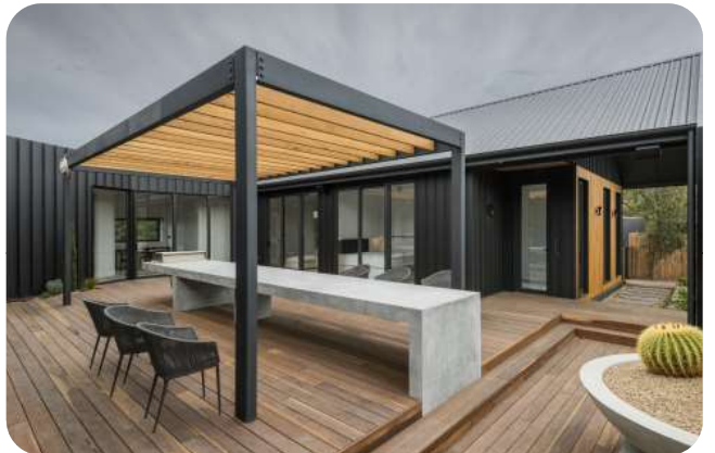
Plate 26 Image: Example of patio height lower than total roof pitch height (from colorbond)
