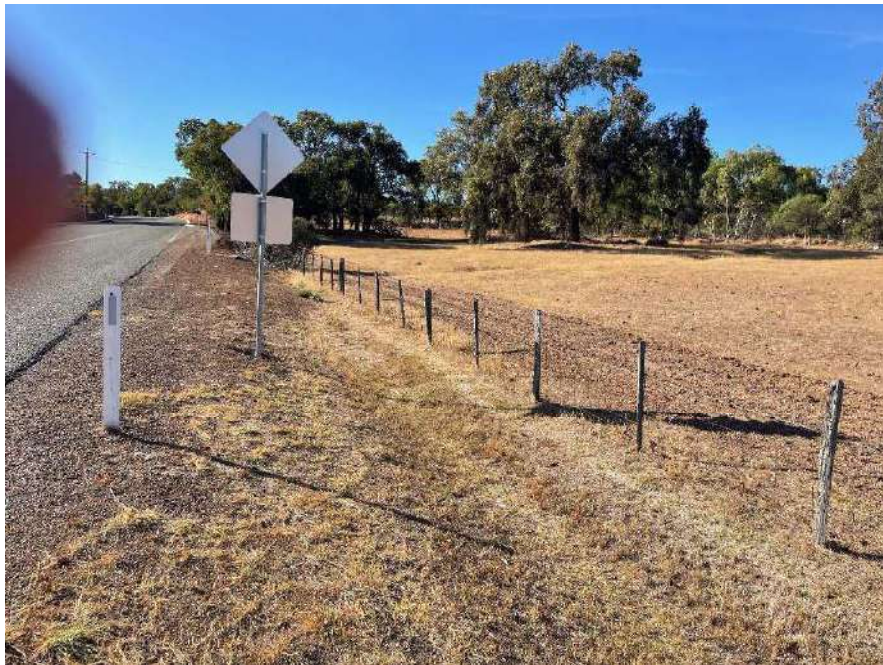
Figure 13: Weld Street roadside swale Photo 4
