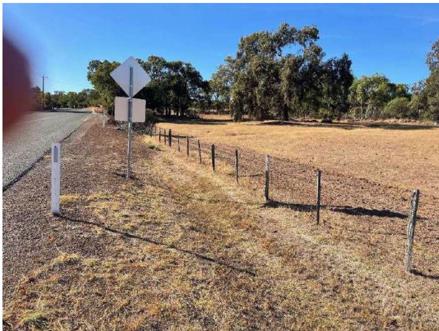
Figure 13: Weld Street roadside swale Photo 4
