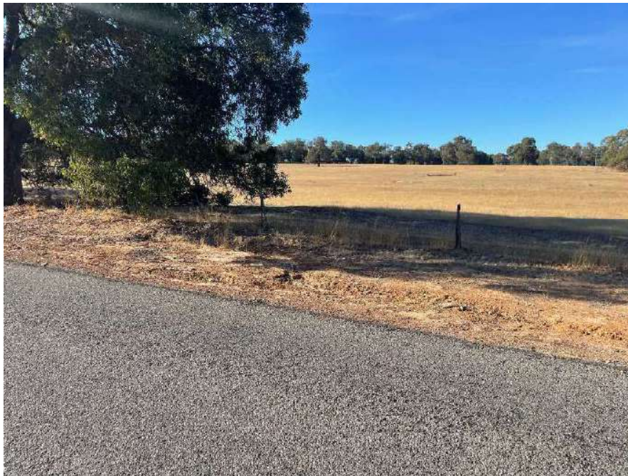
Figure 12: Weld Street roadside swale Photo 3
