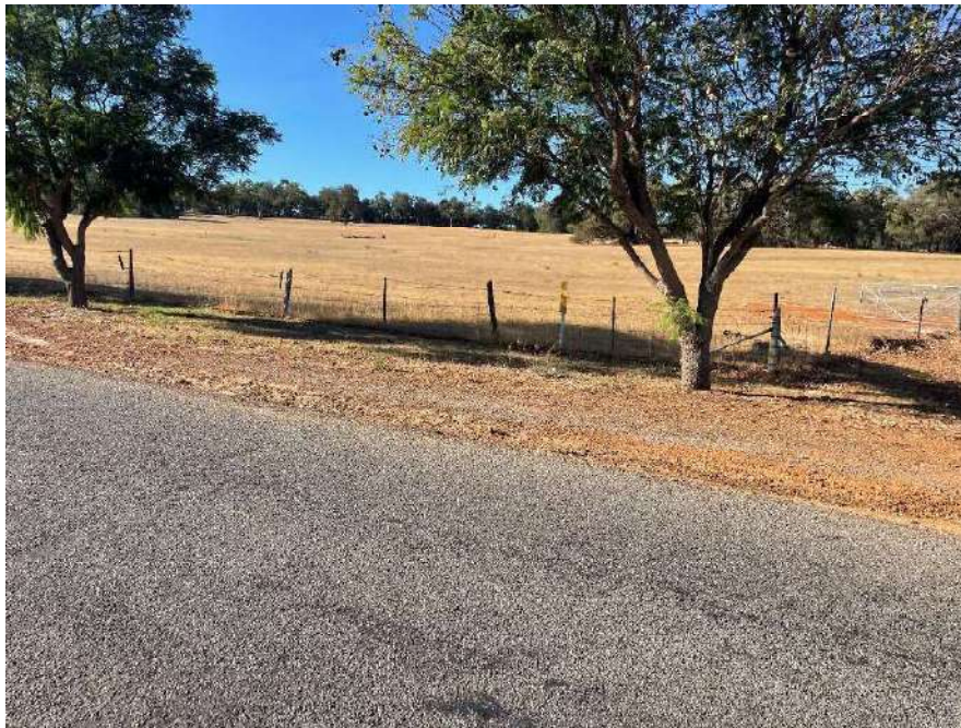
Figure 10: Weld Street roadside swale Photo 1
