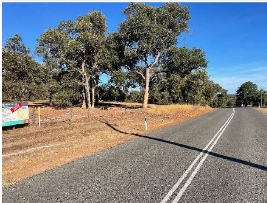
Figure 14: Weld Street roadside swale Photo 5
