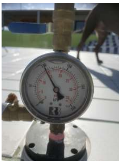
END OF TEST LEISURE
