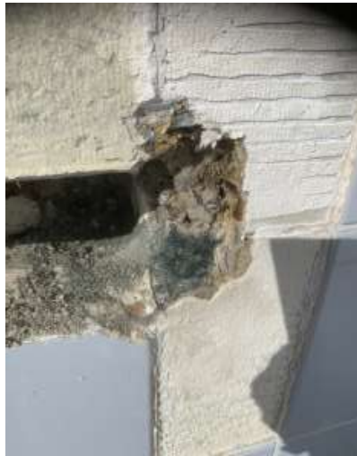
Showing bluey/black colour to concrete due to the pipes in the wall.
