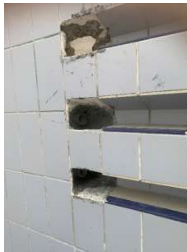
Showing the three steps with exposed pipes
