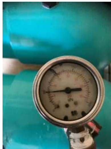
FINISH OF 25 METER TEST
