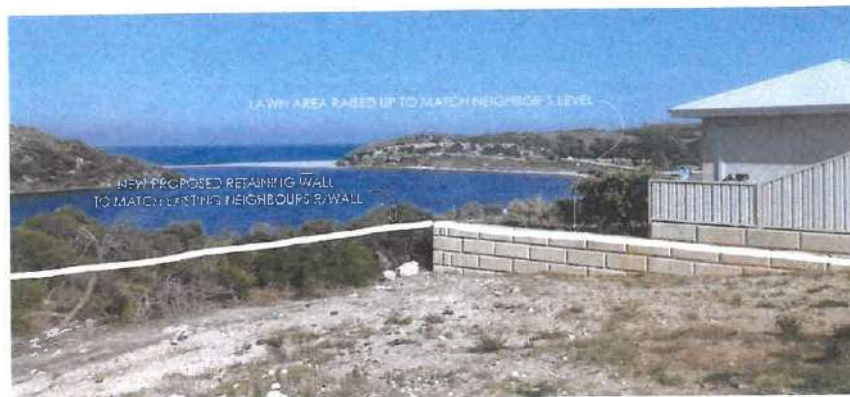
Figure 7 – Proposed retaining wall height to south/west boundary in relation to neighbour
