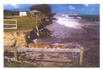
Figure 1: Erosion losses of shoreline in front of Grace Darling Park on 17 May 2015.
