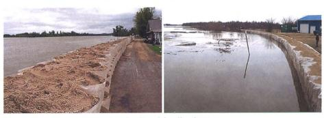
Figure 3.5 **Defencell Barriers for Flood Applications**
