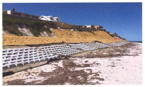
Figure 3.4 Example Concrete Scour Protection - Seabird
