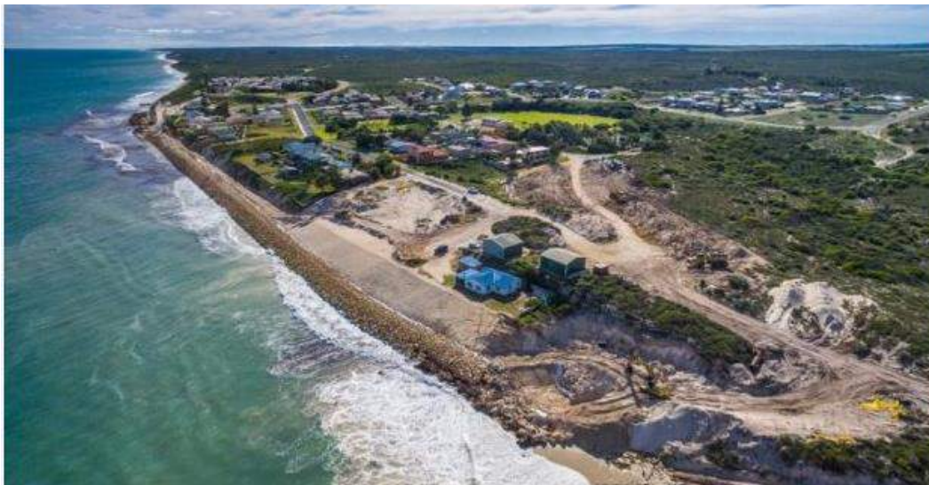
Figure 3-2 Photograph of the Seabird seawall during construction in the SE1 management unit (source, watoday.com.au)
