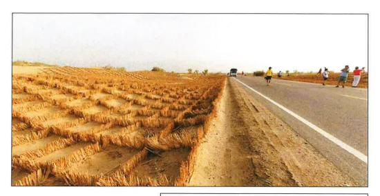
Figure 24. Straw checkerboard technique (DRI 2011) and its application on the Tarim Highway, China (The Tarim Highway, undated).
