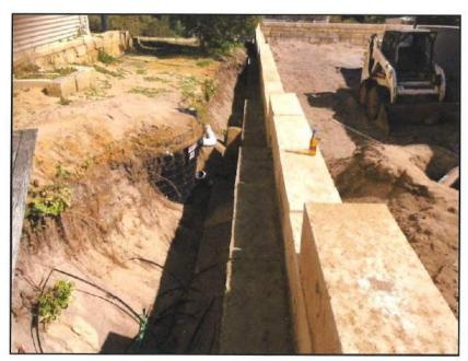
Photo 2: View of the retaining wall footings along eastern boundary
