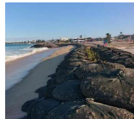
Example: Previous medium term rock bag structure in place at Stockton Beach.
