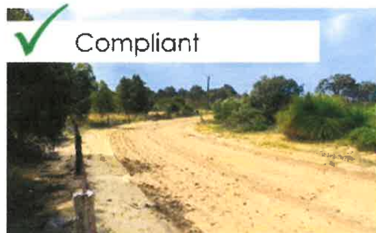
Firebreak is correct width of a minimum of 3m of bare earth
