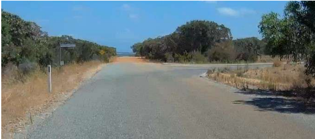
Figure 3.1 Sealed section of Waterville Road, looking west towards Borabilla Place
