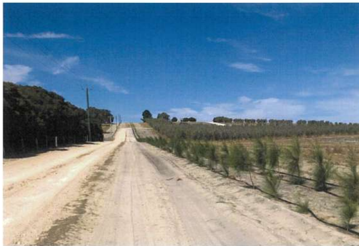
New Casuarina trees with irrigation dripline installed
