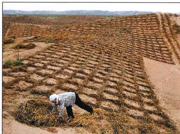
Figure 24. Straw checkerboard technique (DRI 2011) and its application on the Tarim Highway, China (The Tarim Highway, undated).
