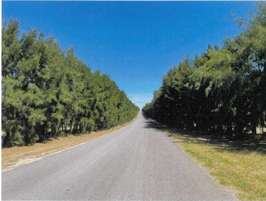
Example of composite bitumen road with Casuarina tree line.
