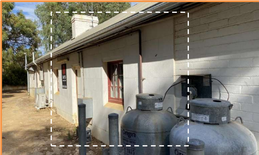
Figure 2b: - Elevation showing Rising Damp
