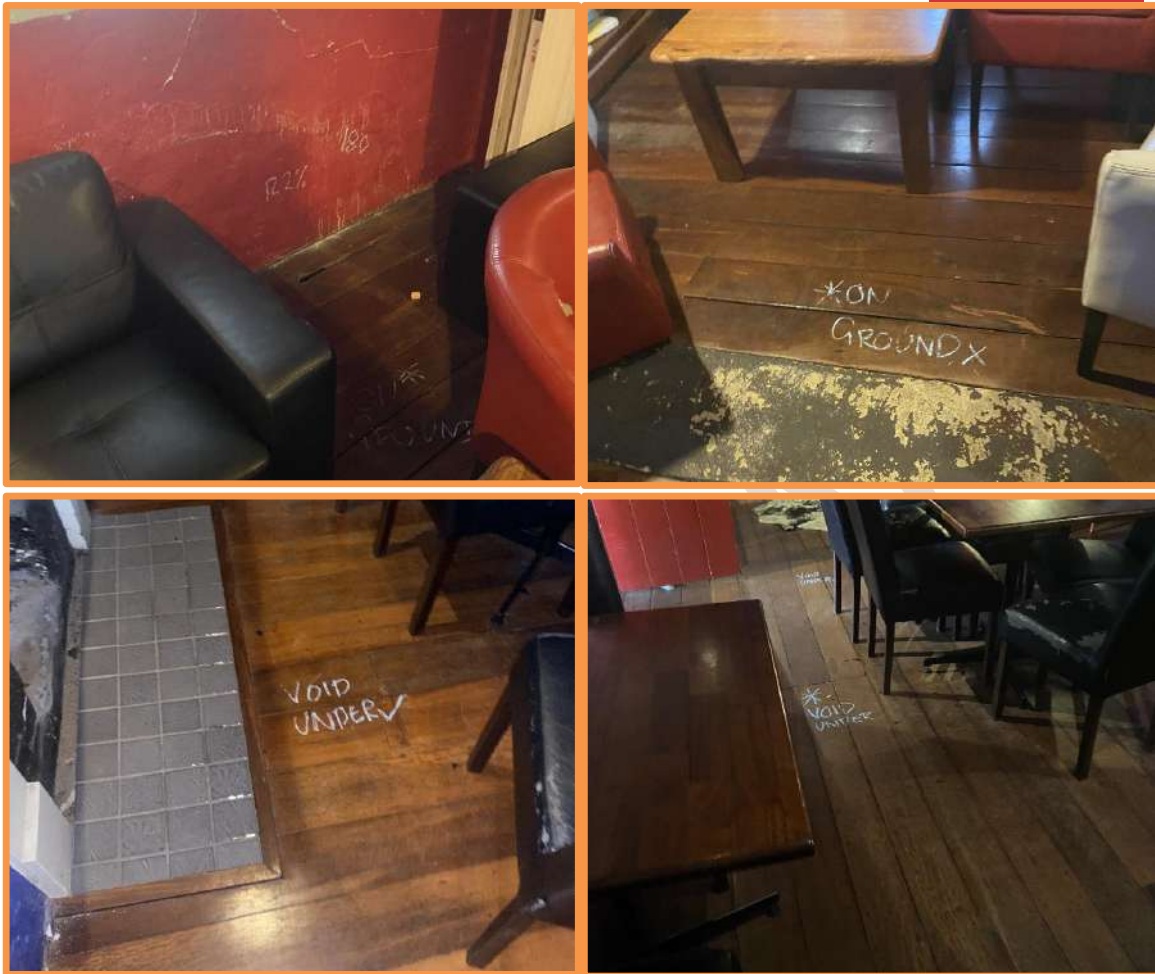
Figure 2k_2: - Existing Floor Support Location
