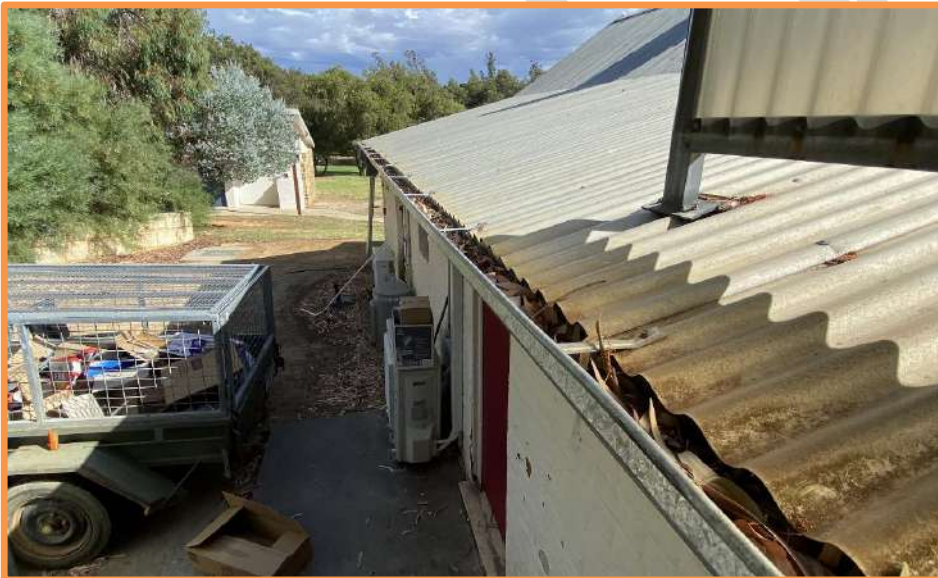
Figure 2h – Clean Gutter of leaf debris
