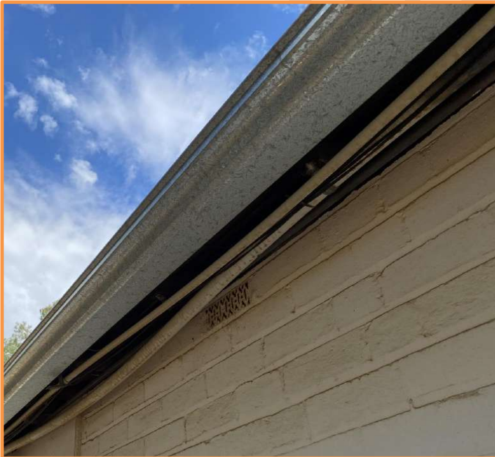
Figure 2c: - Open Gutter and Eaves to Property
