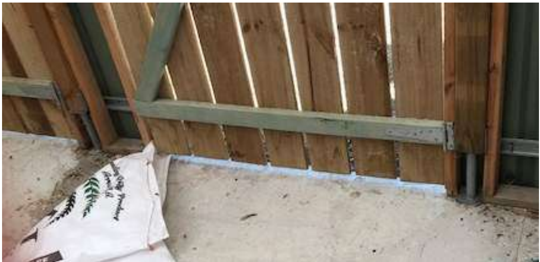
POSTS ON STIRRUPS AT DOORWAYS. CONCRETE FLOOR
