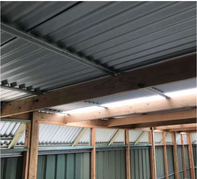
ROOF BATTENS, RAFTERS, EDGE BEAMS TOP PLATE AND WALL BATTENS
