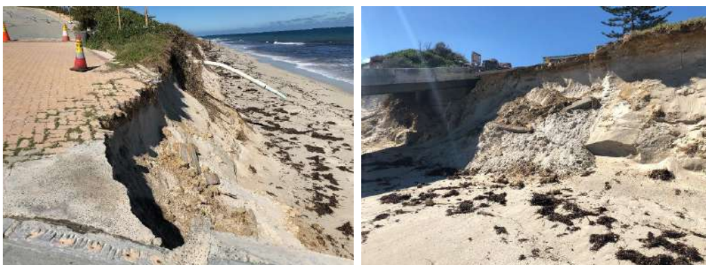
Figure 7 – Beach Access Ramp Erosion on 23/8/18
