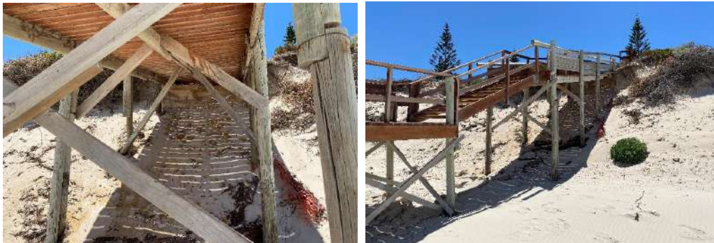
Figure 6 – Nitschke's Walk Erosion Damage on 11/1/22
