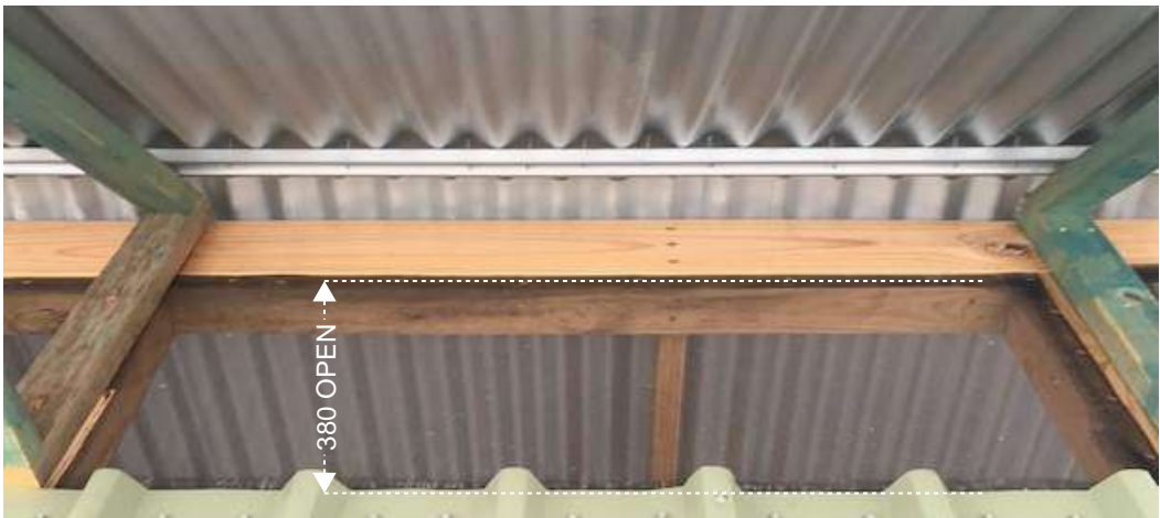
ROOF BATTENS, RAFTERS CONNECTION TO EDGE BEAMS (3 x BUGLE SCREWS THROUGH EDGE BEAM INTO RAFTER END) WALL CLADDING FIXINGS
