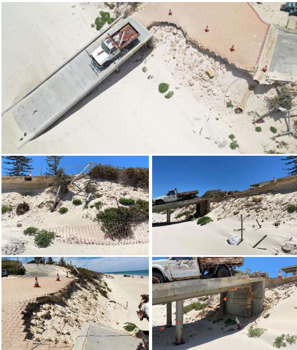
Figure 5 – Beach Access Ramp Erosion Damage on 11/1/22
