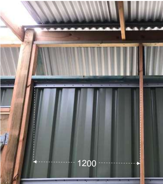
FRAME ATTACHED TO POST. WALL BATTENS. FRAME UPRIGHTS AND SPACINGS
