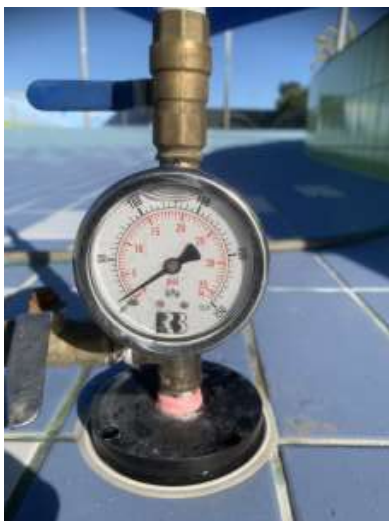
END OF TEST TO FLOOR RETURN THAT NOT CONNECTED
