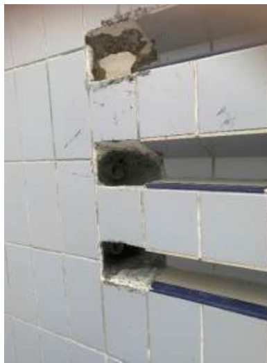
Showing the three steps with exposed pipes
