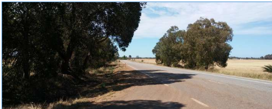
Figure 7: Aurisch Road Looking South
